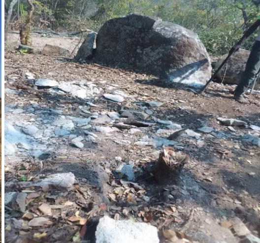
Road clearing in preparation for the rig to pass
